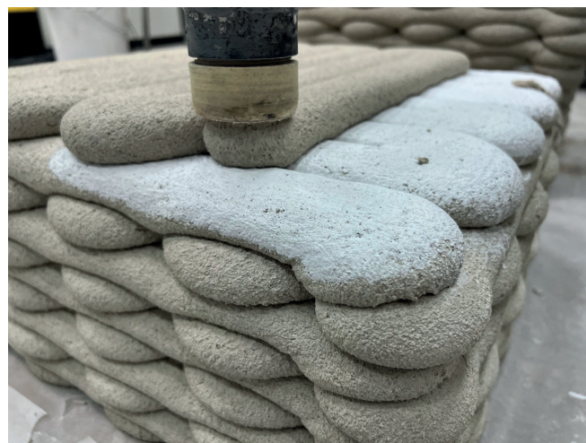
Figure 9. Printing process over a processed cold seam
