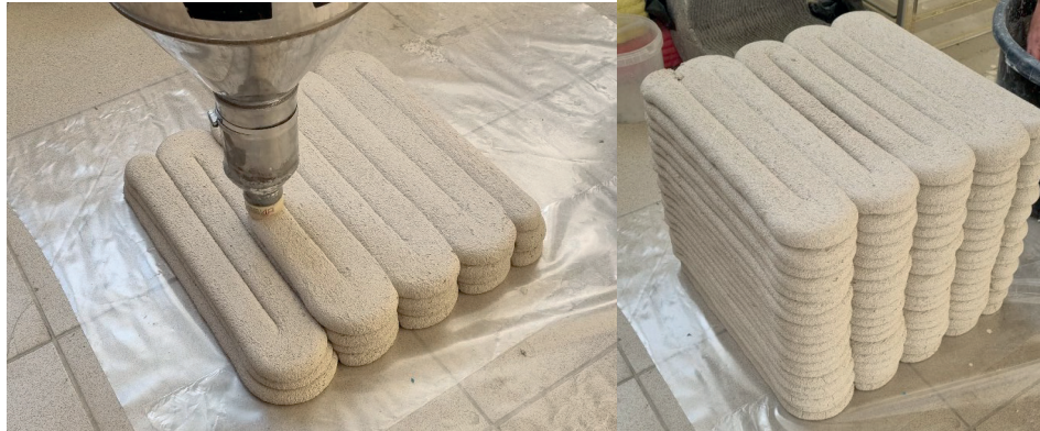
Figure 5. Printing of a parallelepiped-shaped product with layer-by-layer laying of the mixture in one direction and the appearance of the finished product
